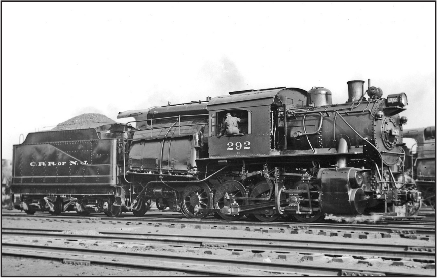
Central Rail Road of New Jersey, #292, a 0-8-0. So you want to drive a camelback? Camelback's wide fireboxes restricted driver visibility to the rear. – Photo, Tom Klinger collection.
